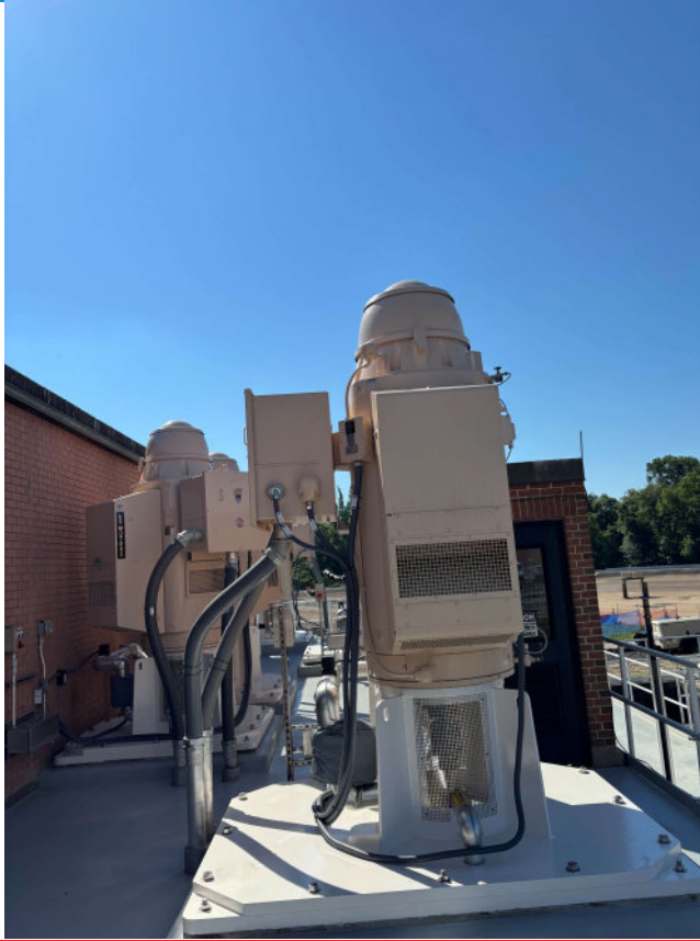
Secondary Effluent Pumps Replacement
