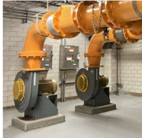
Combustion Air Blower
