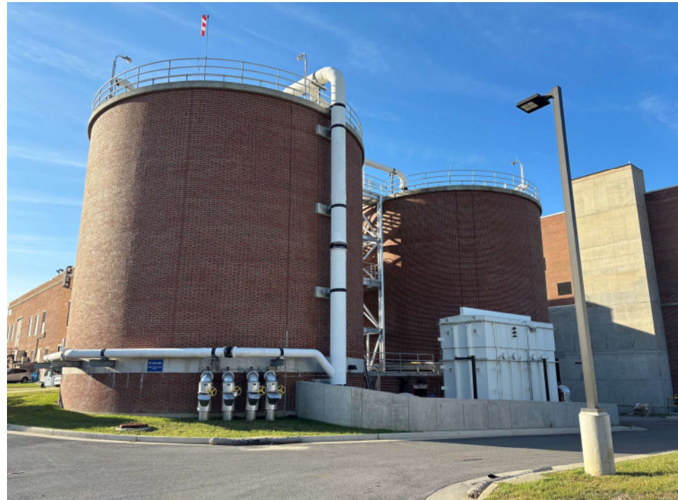
Sludge Storage Tanks
